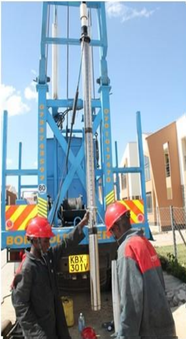
Test Pumping System/ Installation Team
