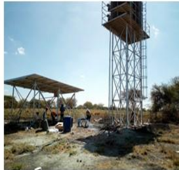
Solar pumping systems
